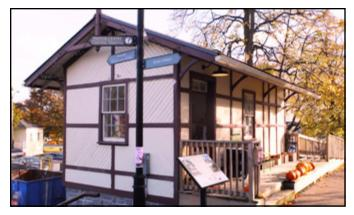
The current project is replacing the old asphalt roofing with eastern cedar shingles on a repaired wood structure and roof deck. In addition other minor wood repairs have been made where pests, birds, and squirrels had made openings in the siding, and the building is being repainted. This repair and maintenance work should stabilize the building for many years to come.
